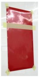
2. Place a horizontal strip of tape across the decal, 100 to 200mm down from the top edge, as a hinge. Place further sections of tape along all sides 300 to 500mm apart that will act as registration tabs during application.
