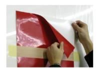
3. Separate the upper portion of the liner from the graphic and remove this section of the liner by cutting it with a snitty or knife. Use the knife at an angle to avoid cutting into the wall surface or the graphic.
