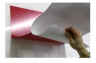
6. Reach behind the graphic and carefully pull the liner back several inches to expose the adhesive.
