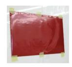
Measure and position the graphic using masking tape to hold it in place. It is a good idea to mark the position of the panel in case the graphic comes loose. Wherever possible make sure the graphic is completely smooth and taut.
