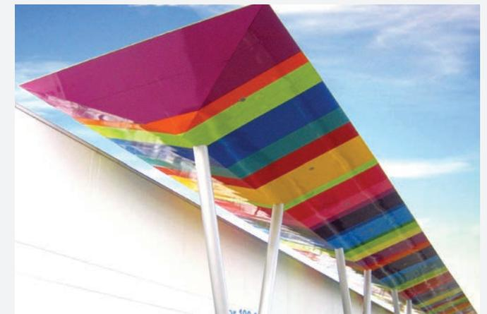
**900 Super Cast** High gloss, premium vinyl with improved durability for outdoor applications. It is an extremely conformable film suitable for irregular surfaces and complex applications including heavily corrugated surfaces, convex and concave curves.
