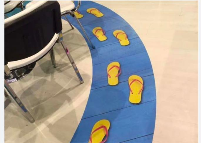
**Mactac FloorGrip** overlaminate is a non-slip protection film that is conformable on difficult surfaces such as tarmac, bitumen and stone. You can ensure your floor graphics are well protected from UV and abrasion, even in high traffic areas.
