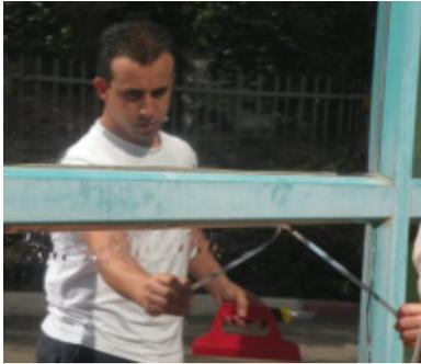
**Step 10** - Trim the edges of the film adjacent to the window frame, using the sharp knife and the Edge Tool.
