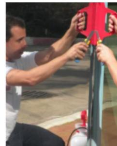
**Step 9** - Using a 6" heavy-duty safety film squeegee, wipe from the center with firm downward and outward movements, removing water and air bubbles trapped between the film and the glass.
