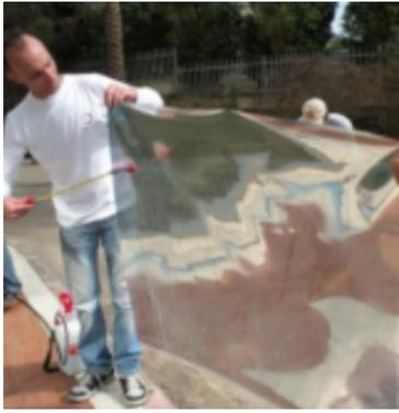
**Step 4 - Spray film:** Spray film on both sides to avoid static (less dirt in installation) and flatten the film.
