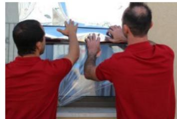
**Step 8 alternative** - The two installers position the film on the window with the wet adhesive side on the glass. While one installer supports the rolled film, the other pulls the release liner downwards from beneath.
