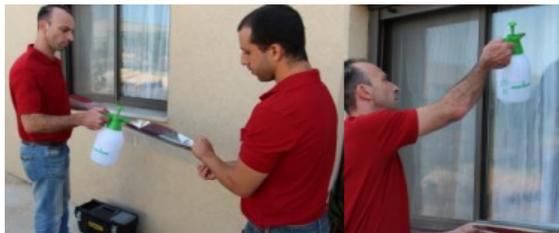
**Step 7 alternative** - Separate release liner from the precut film (rolled with liner outside) and spray the exposed adhesive layer generously with wetting solution. Make sure to wet the window with plenty of wetting solution!
