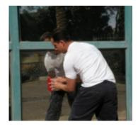
**Step 12-** Wet the film surface again, and pressing hard with the squeegee, wipe out from the center until all the air bubbles and remaining water has been removed from the edges.
