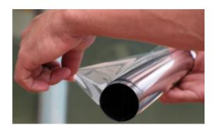
**Step 3 - Precut film:** Precut film to window size, leaving 2cm overlapping edge all around: prepare the film straight from the box, cutting from the hardcoat side with a sharp blade. Make sure the film is rolled with a release liner outside (SR coating inside).
