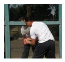
**Step 8 -** Position the film on the window with a wet adhesive side on the glass.
