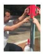
**Step 10 -** Trim the edges of the film adjacent to the window frame, using the sharp knife and the Edge Tool.
