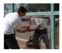
**Step 9 -** Using a 6" heavy-duty safety film squeegee, wipe from the center with firm downward and outward movements, removing water and air bubbles trapped between the film and the glass.
