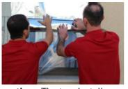
**Step 8 alternative -** The two installers position the film on the window with the wet adhesive side on the glass. While one installer supports the rolled film, the other pulls the release liner downwards from beneath.
