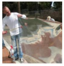
**Step 7 -** Remove the release liner from film and spray the exposed adhesive layer with plenty of wetting solution.
