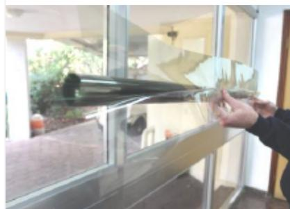
2. Spray both sides of the exposed 6 inches with the wetting solution.
