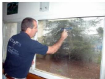
13. Trim the edges of the film adjacent to the window frame, using an Olfa knife and if needed you can use a straight-edge as an edge guide
