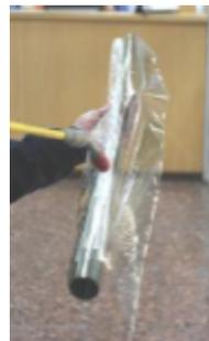
4. Spray the exposed adhesive layer with plenty of wetting solution on the clean glass.
