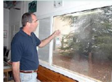
6. If the installation is taking place in an extremely dry region it may be necessary to wet the film on both sides (get help from another person at this stage) to reduce static. Rewet the glass surface.
