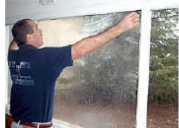
3. Cut the film to the size of the window, leaving  $\frac{3}{4}$ " (2 cm) overlapping edges all around. Alternatively, measure the window and pre-cut film out of the box or on a Film Handler.
