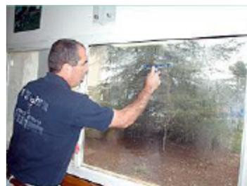
15. Wrap a lint-free paper towel around the edge of the hard card and "bump" around the edge of the installed film. Wipe dry the edges of the film and the window using paper towels.
