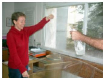
9. Place the wet adhesive side of the film onto the glass.
