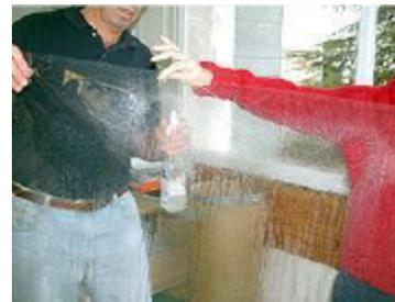
7. Using two pieces of adhesive tape, separate the backing liner from the film removing the liner completely
