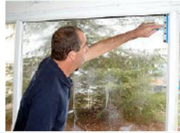
5. Re-wet the window, using plenty of slip solution.
